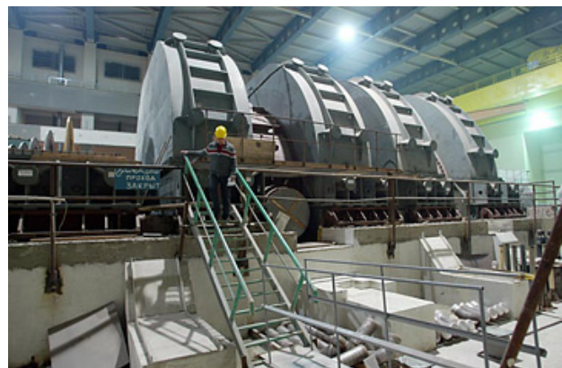
The Bushehr nuclear power plant
