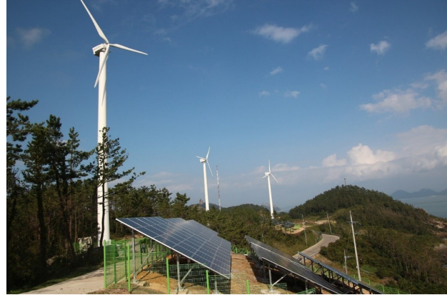
Wind turbines and solar panels used in Microgrid on Gasa Island: Courtesy of KEPCO.
