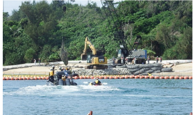
A protester on a kayak approaches Henoko construction site, May 15, 2017. Photo: Tsuyoshi Kitaueda
