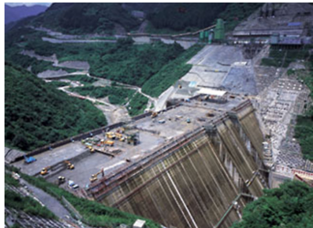
Takizawa Dam, second construction
