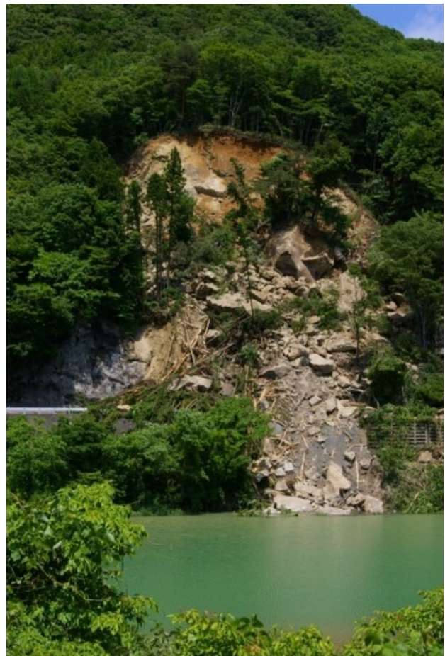
The Iwate-Miyagi Nairiku Earthquake
