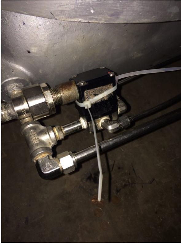
**Photo from an inside source reveals the solenoid bypass which led to the June 2016 leak**
