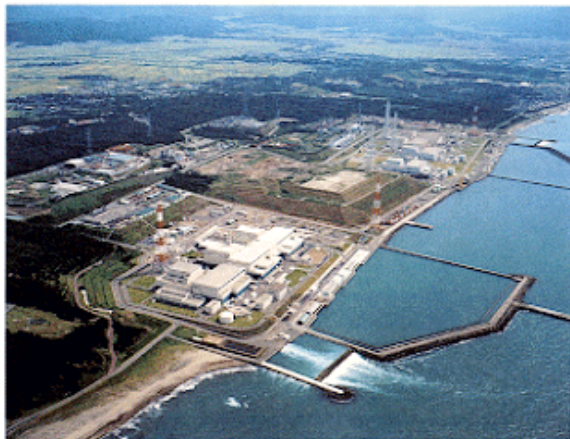
The Kashiwazaki-Kariwa plant
