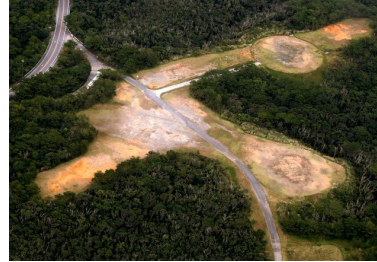
Gouged Forest and Completed "Osprey Pads" Asahi shinbun December 17, 2016.
